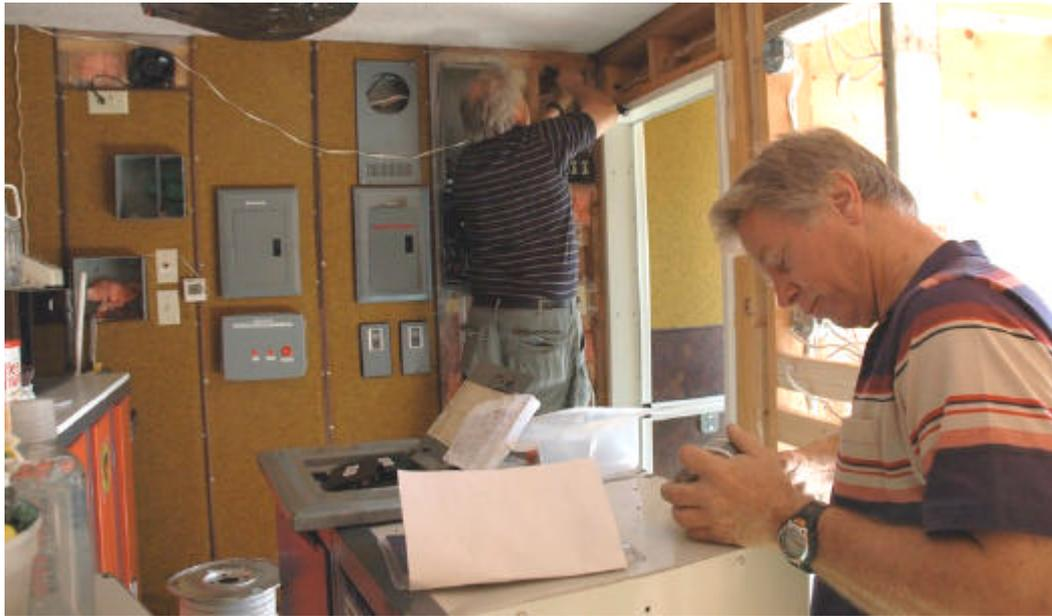
Renovations to the Sleaford Observatory warm-up shelter progressed rapidly last fall with Rick Huziak and Darrell Chatfield spending many days and evenings there. A wall was removed to the cold storage area to make more room, which meant extensive rewiring, insulating and refinishing. Other volunteers came to cut grass, paint, clean, do repairs, and provide food. Thank you to every one who helped to make Sleaford a more usable and pleasant site.
